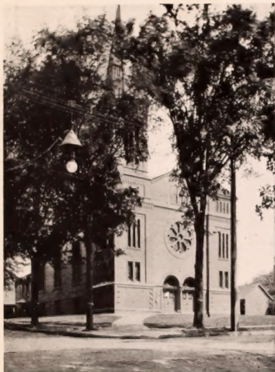
Congregational Church Woburn Street, Reading, Mass.
